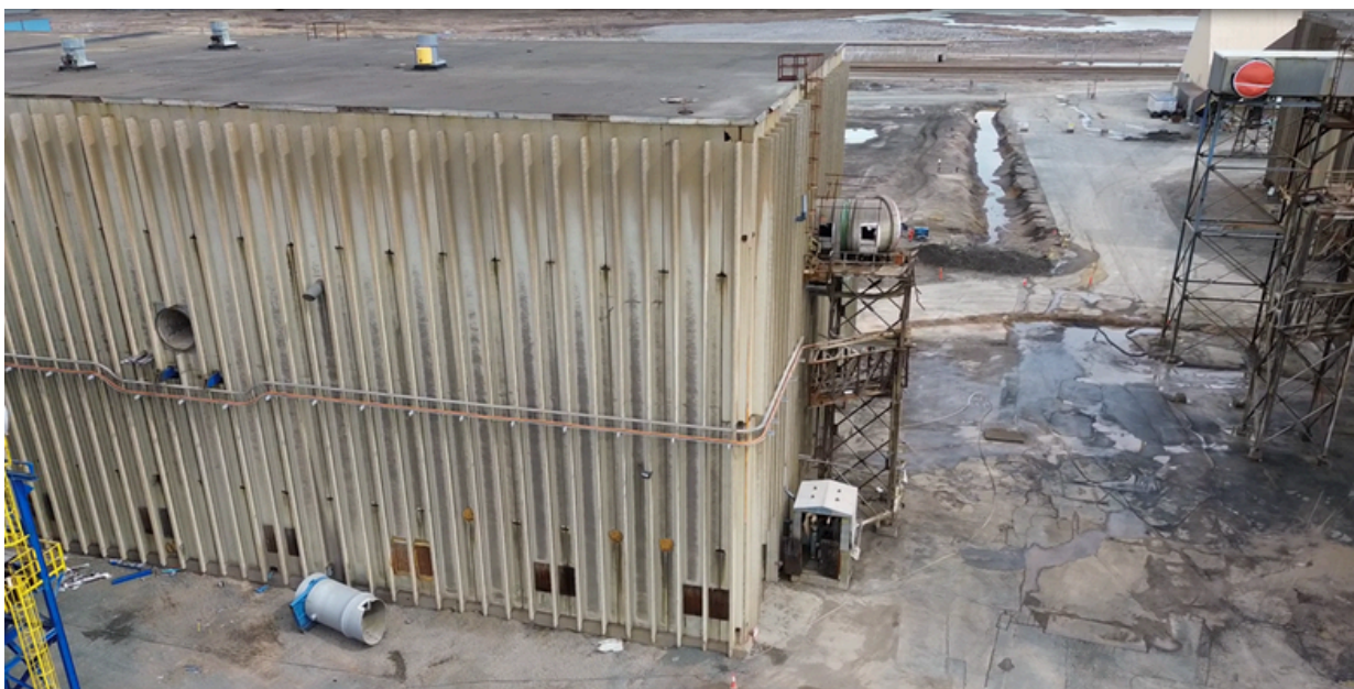
Clean-up following Hot Gas Precipitator outlet duct removal
