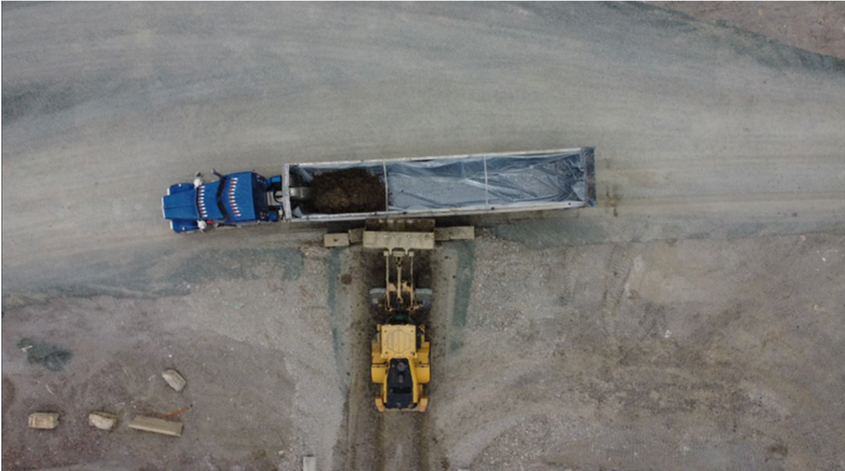
Loading trailer for transportation of materials to off-site disposal facility
